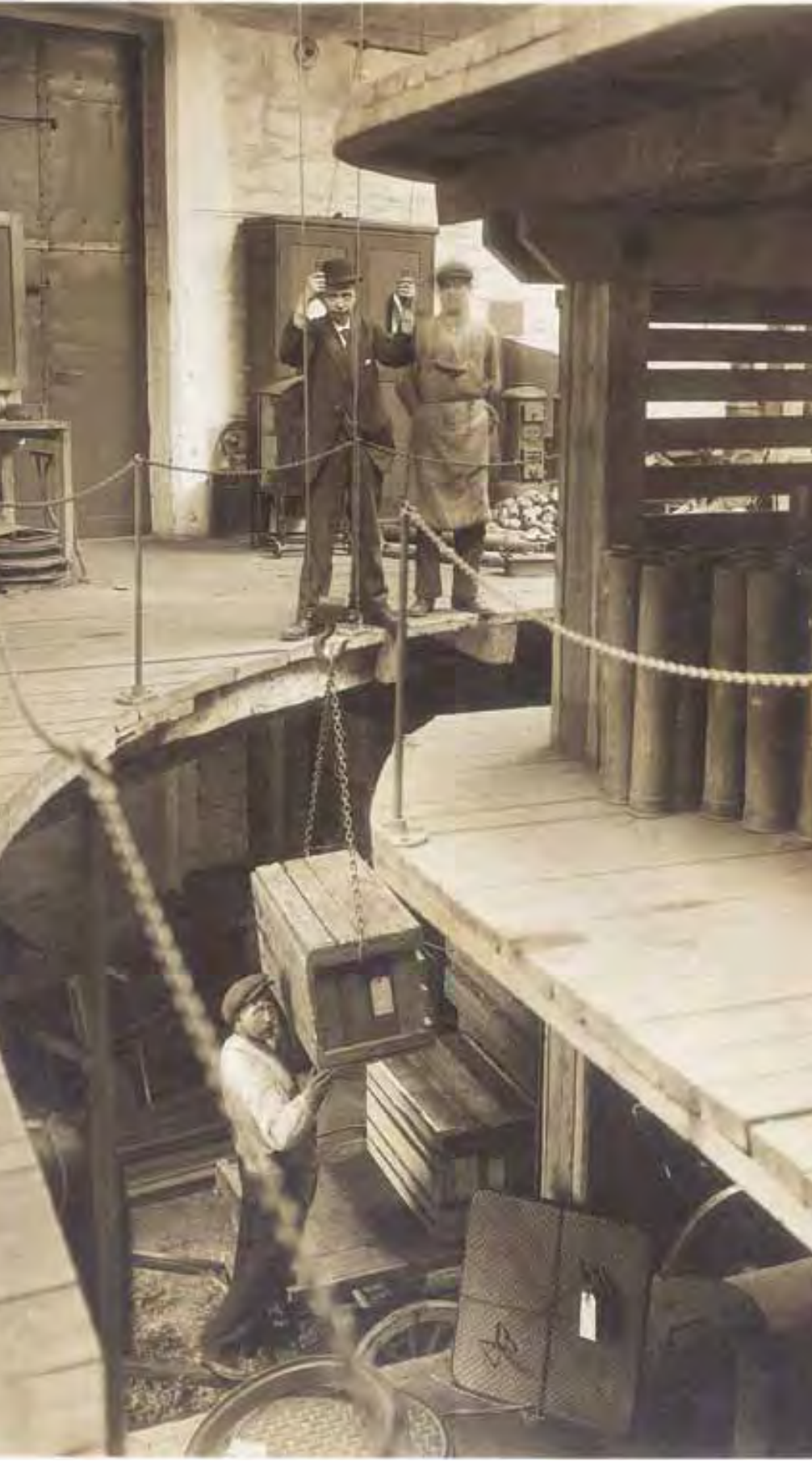
Receiving at the Kværner Works foundry. The photo is from around 1900 and shows that transport was still done with muscle power. In the lower story a horse and cart can be seen. From there the goods were hoisted up manually with block and tackle.
