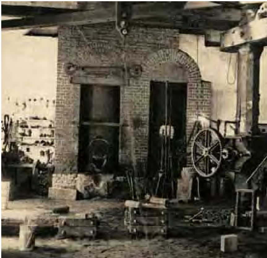
Cupola furnace at Fritzøe Works in Larvik, erected around 1850. The picture was taken almost 100 years later, but still gives a good impression of how an early Norwegian iron foundry looked. The foundry was used almost exclusively for the company's own purposes, and was thus not greatly modernised during its lifetime.
